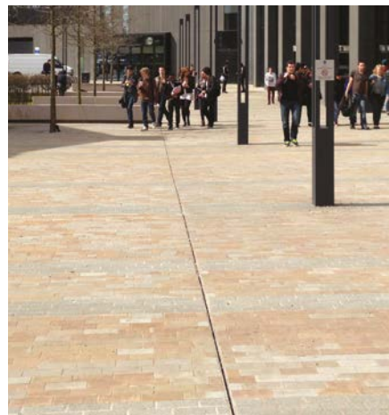
Warm coloured mix of natural coated concrete paving to thoroughfare sections
