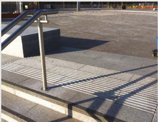
Handrails and contrasting nosing on steps
