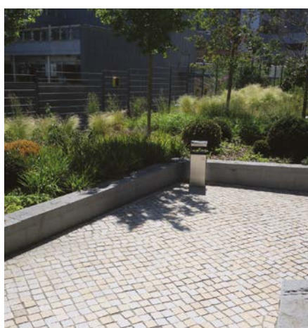
Collegiate Courtyards - Tumbled sets, detailed pattern and tonal colours, used in conjunction with accessible materials
