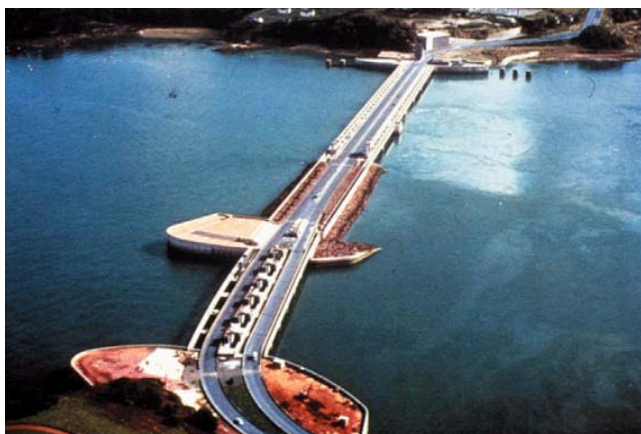
La Rance tidal barrage operating successfully for over 40 years
