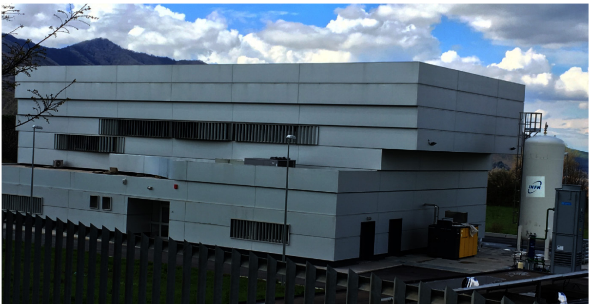
Test facility Thor at the University of Salerno.
