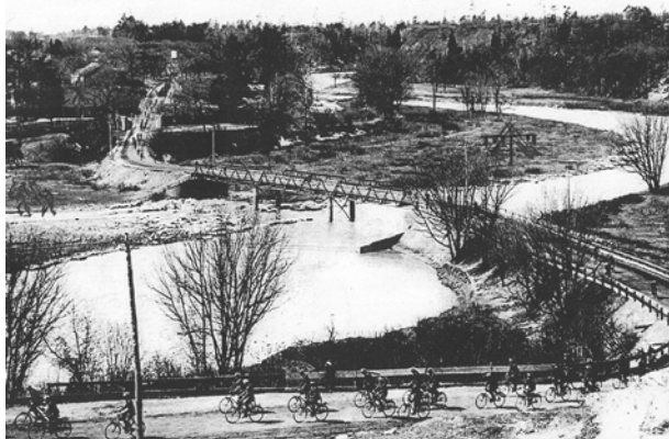
Figure 3: Archival photo of WWI Cycle Corps training at the Humber River. 1914.
