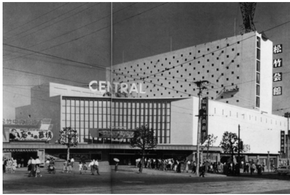
Figure 3, Shochiku Hall, 1962, Cinema theater as a landmark.
